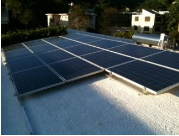
PV Solar 4 KW system in Manati
