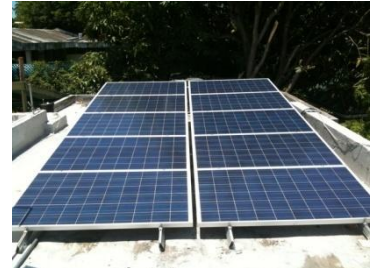
PV Solar 2.2 KW system in Guaynabo
