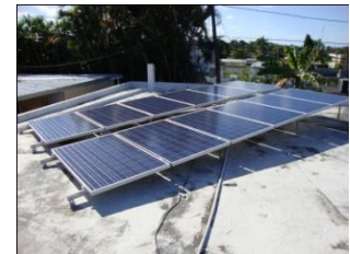
Solar/Wind 3.6 KW system in Rio Piedras
