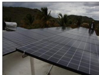
PV Solar 4.4 KW system in Salinas
