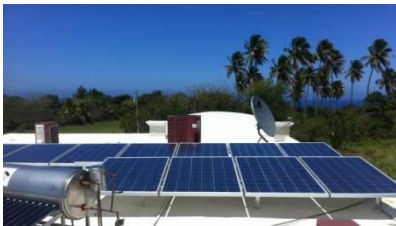
PV Solar 2.4 KW system in Isabela
