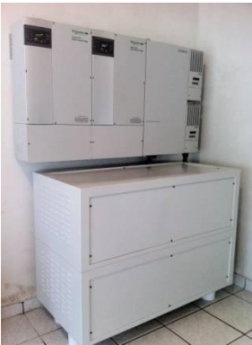
PV Solar 8 KW system with SolarMax battery cabinets in San Sebastian
