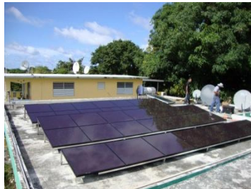
PV Solar 3 KW system in Hatillo
