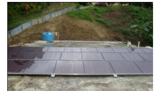
PV Solar 1.8 KW remote system in Patillas
