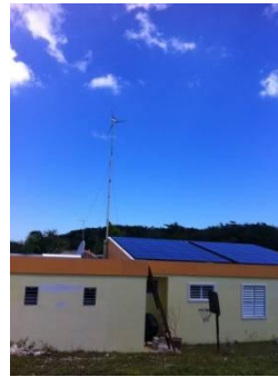
Solar/Wind 4.2 KW system in Aguadilla
