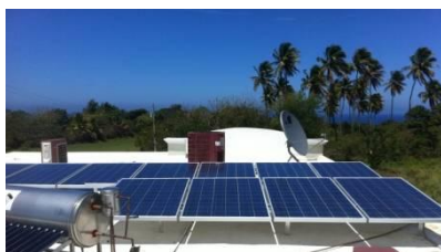
PV Solar 2.4 KW system in Isabela
