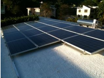
PV Solar 4 KW system in Manati
