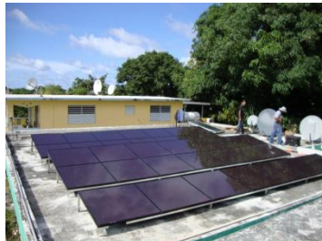
PV Solar 3 KW system in Hatillo
