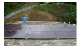
PV Solar 1.8 KW remote system in Patillas
