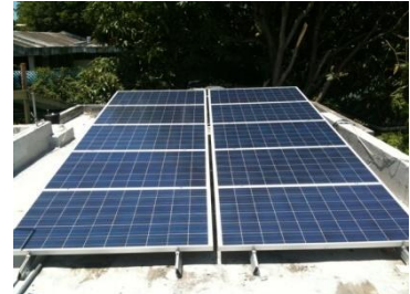
PV Solar 2.2 KW system in Guaynabo
