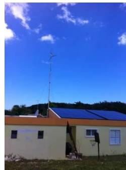
Solar/Wind 4.2 KW system in Aguadilla
