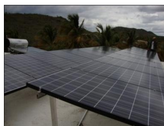
PV Solar 4.4 KW system in Salinas
