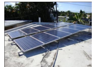
Solar/Wind 3.6 KW system in Rio Piedras
